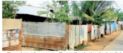
Chunnakam refugee camp: The small rusty zinc sheet-roofed homes that house 112 families. Pix by Indika Handuwala
